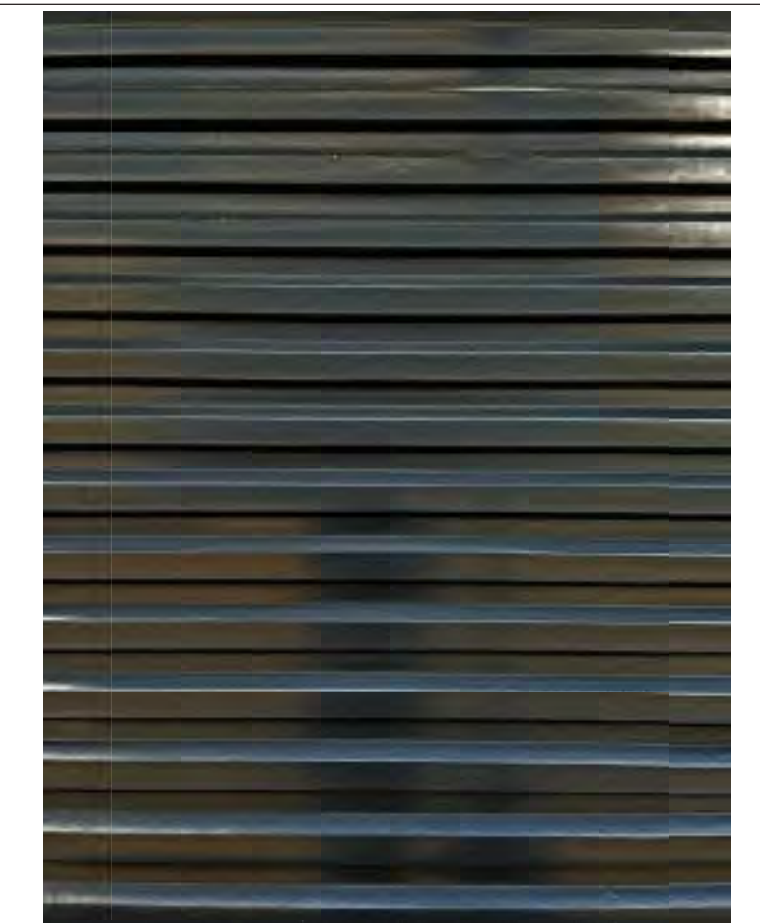
5 TYPICAL RIBBED METAL WALL PANELING (MP-1)
